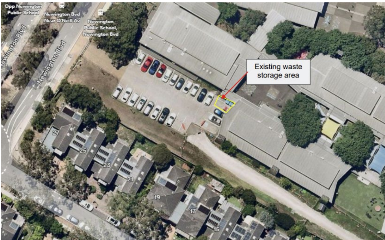
Figure 20: Existing waste storage area (Source: MRA Consulting Group)
